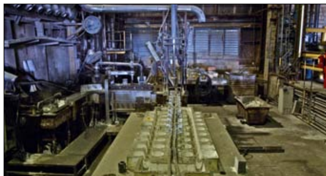
Figure 3. The casting pit with Wagstaff casting tables and NuMax tooling.
